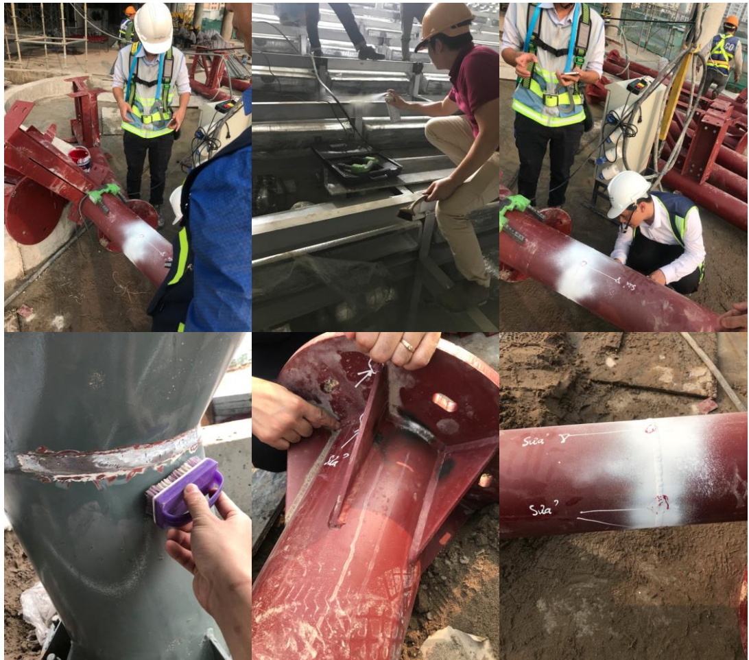
Figuer 2.Ha Noi City RR3 construction project ( Mai Dich - South Thang Long section )
